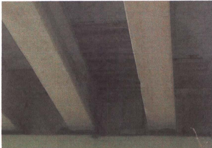
PLYWOOD IN PLACE AT PIER 'A'
